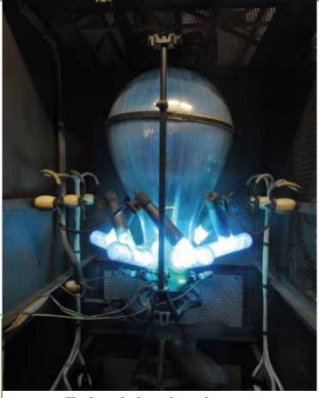
The funny-looking object above is a mercury-arc rectifier, one of the last working in the world which, until recently, powered the trams of the Manx Electric Railway. The apparatus is about a metre high. This is one of the photographs we didn't use in Power, Poles & Platelaying
